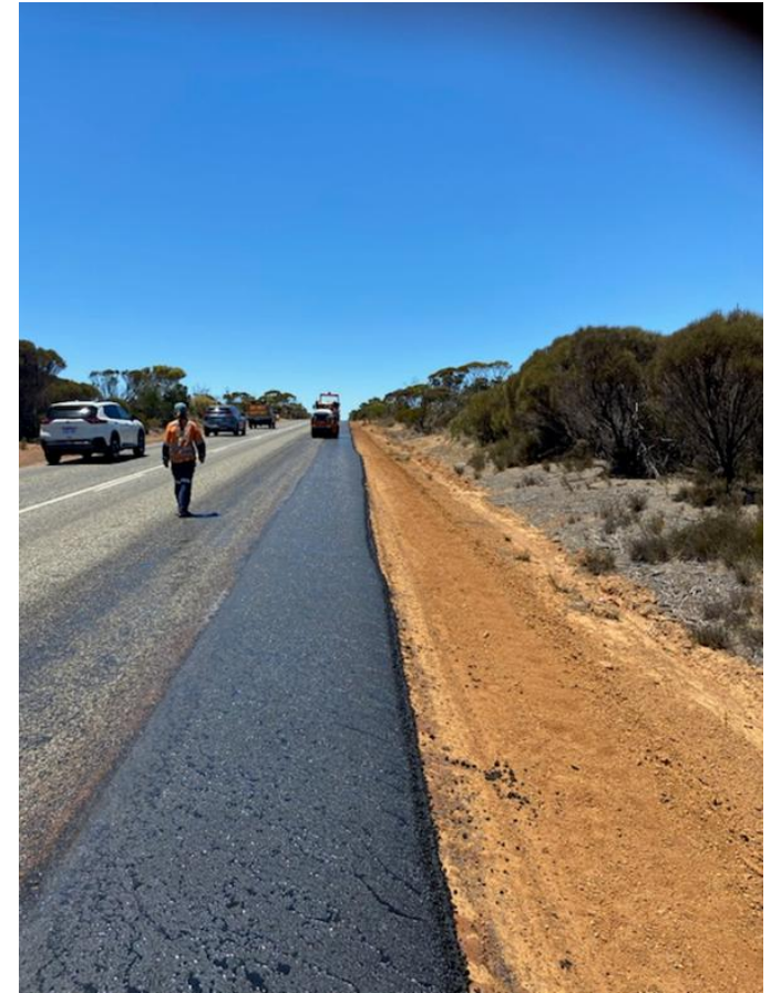
Asphalt widening Collie – Lake King
