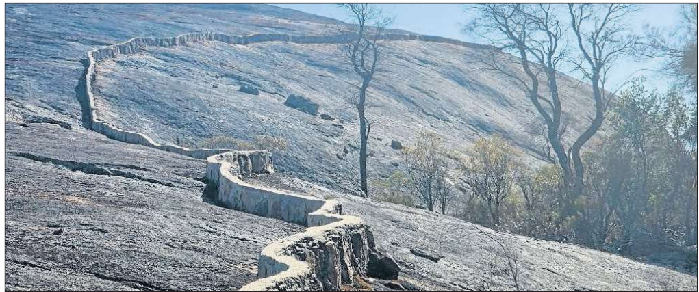
□ Built over about 12 hectares of rock, Pingaring's cement catchment wall guides water into the two-million gallon concrete storage tank, through troughs, open drains and a main pipe.
