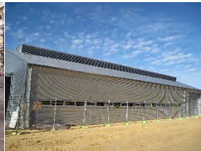
Pattern Shop Extension
